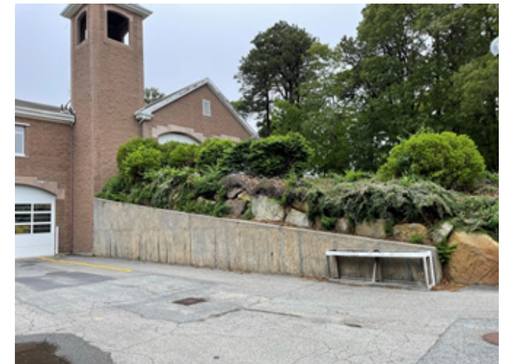
Photo #8 North Retaining Wall
