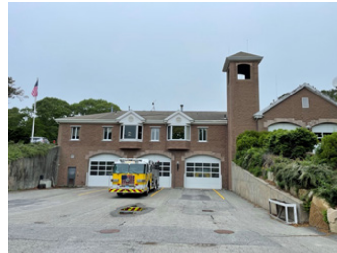
Photo #7 Building East Elevation Hose Tower and the Main Apparatus Garage Doors at the basement level
