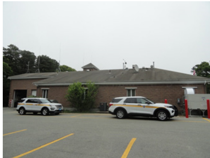
Photo #2 Building West Elevation
