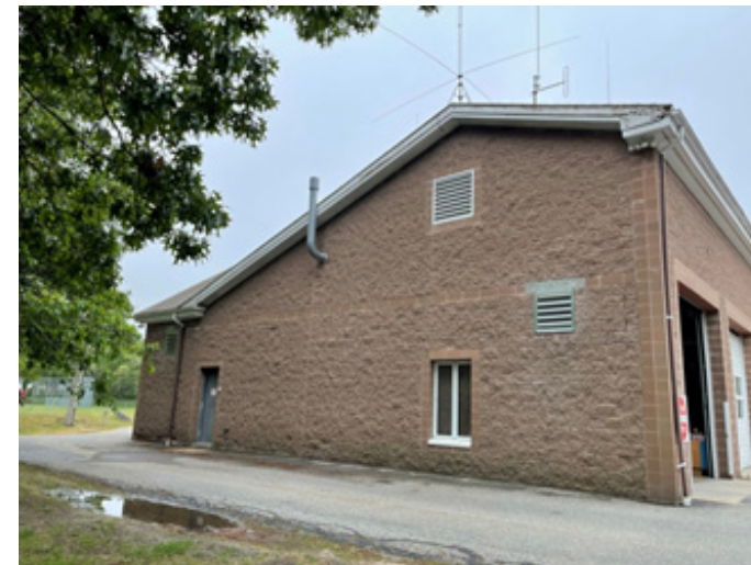
Photo #5 Building North Elevation
