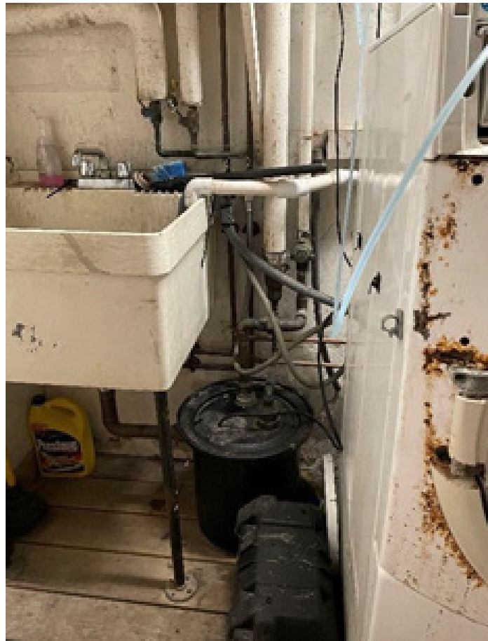
Ejector Pump for Laundry Tub
