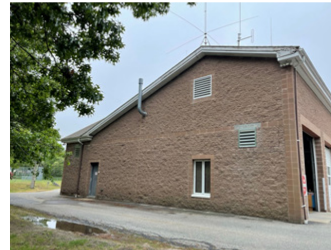
Photo #5 Building North Elevation
