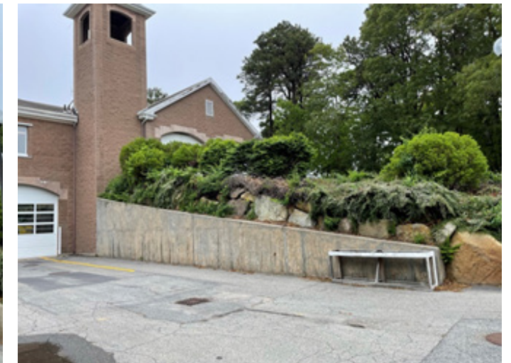
Photo #8 North Retaining Wall
