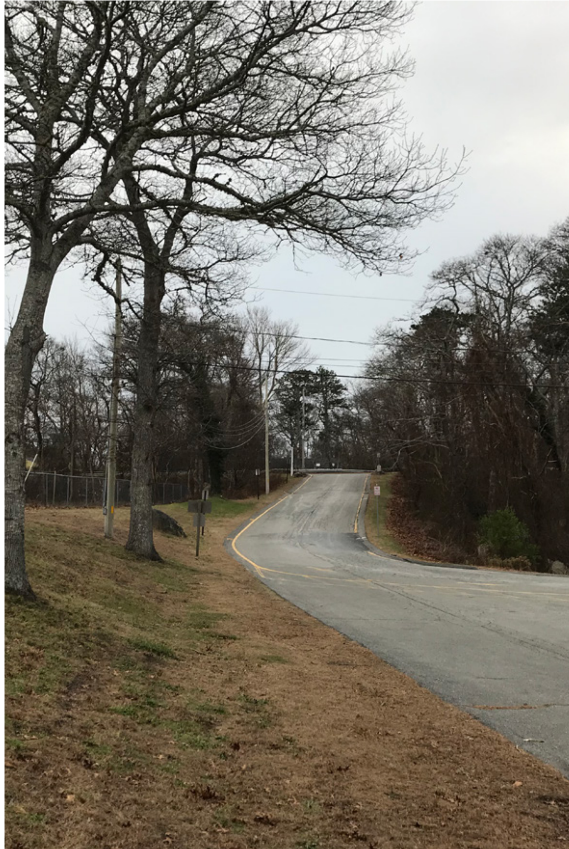
Significant grade changes causing slow turnout time in winter storms
