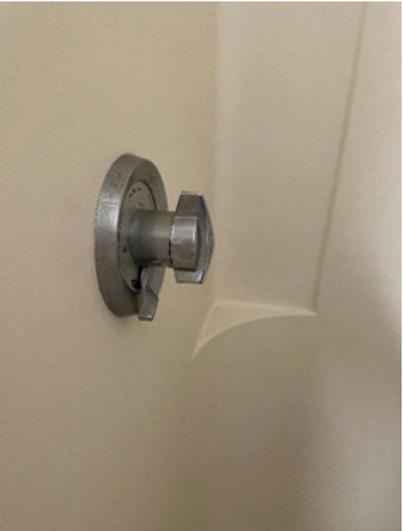
Existing Shower Valve
