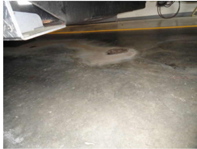
Photo #10 Basement Apparatus Room slab Shrinkage cracks at the front north bay
