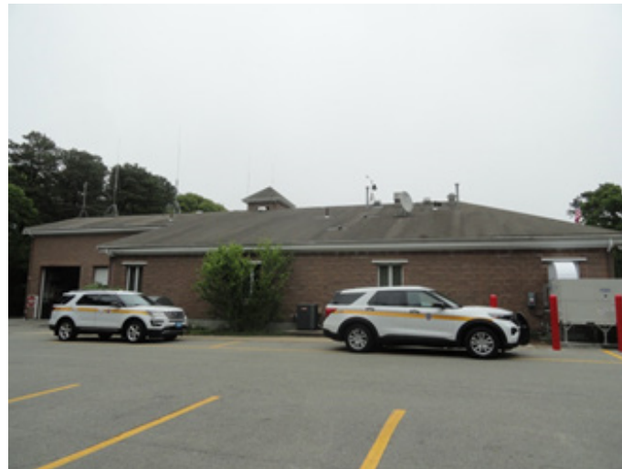
Photo #2 Building West Elevation
