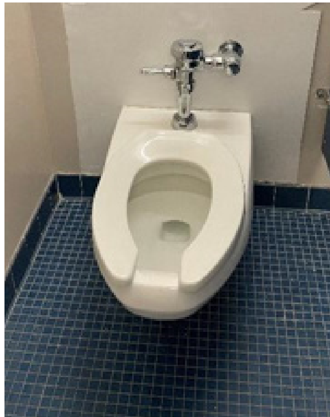
Existing Water Closet
