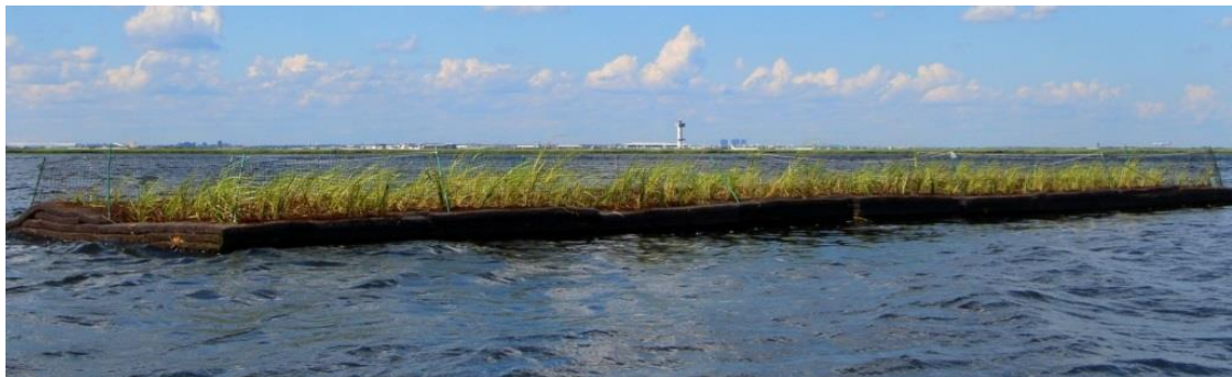
Jamaica Bay Floating Wetland Wave Attenuator
