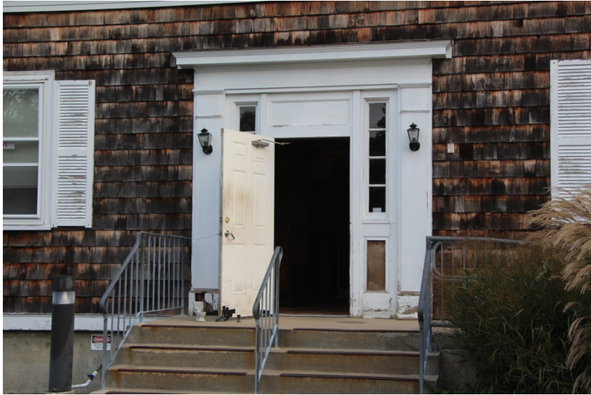
Admin Building Siding and Trim
