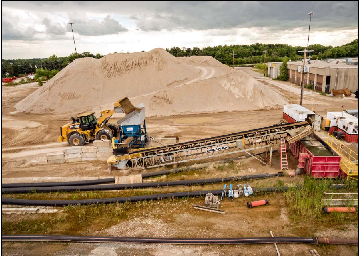
Figure 32. 50,000 CY stockpile of dewatered, dredged material.
