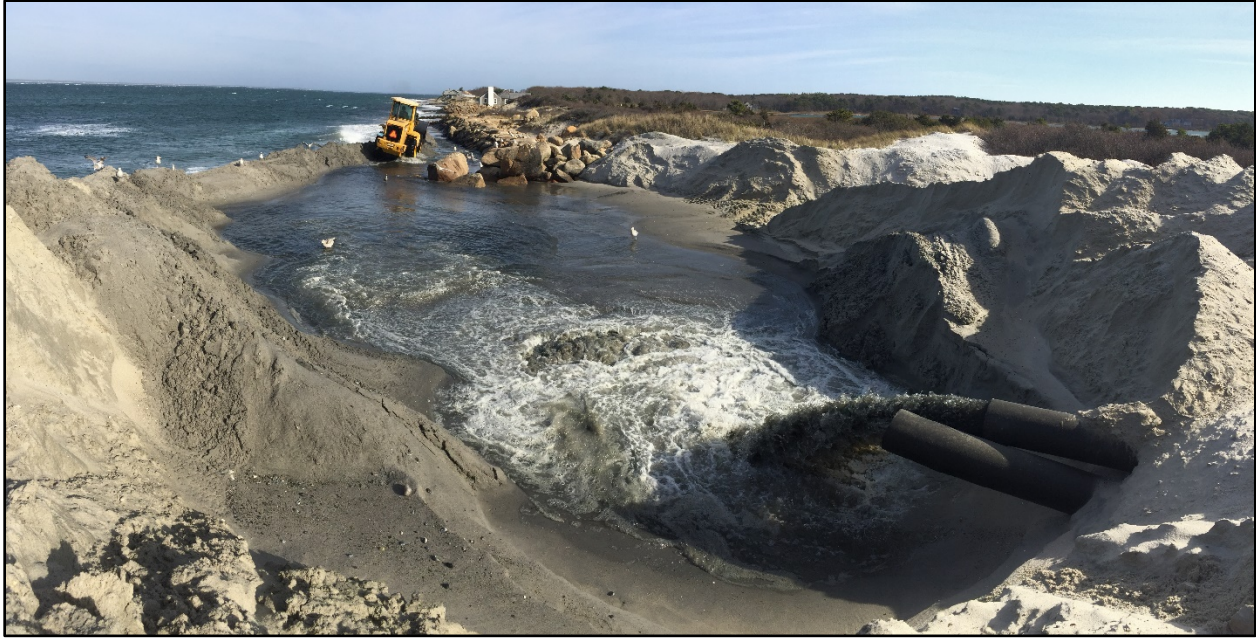
Figure 4. Edgartown Municipal Dredge discharges dredged material at dewatering site. Dewatered material is then stockpiled for beneficial reuse, November, 2020.
