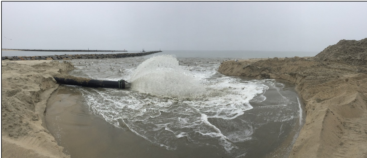
Figure 16. Active BCD dewatering site on Cold Storage Beach, Dennis during operations in Sesuit Harbor, February 13, 2020.
