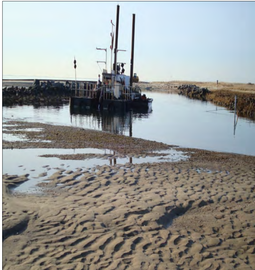
Chatham's south coast shoreline dredging project at Mill Creek Mill Creek.
