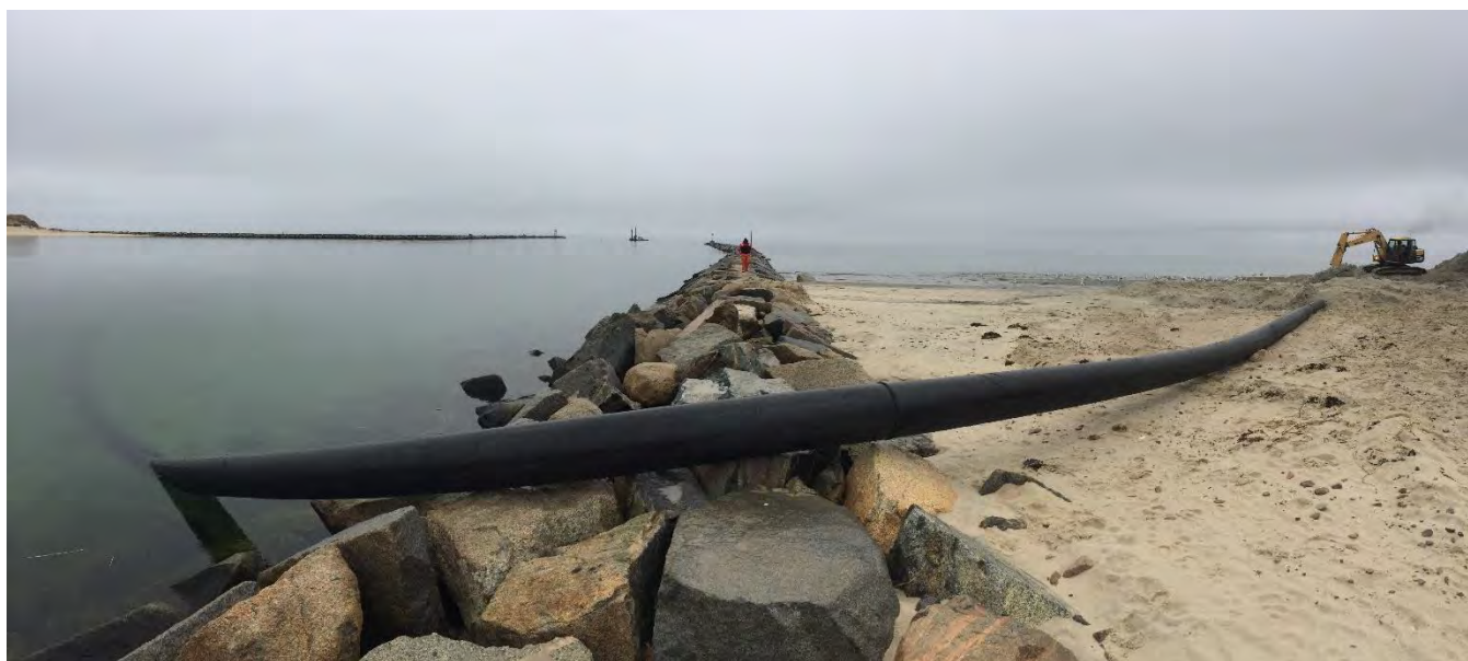
Figure 4 – Dredge pipe comes ashore, Cold Storage Beach, Dennis, MA.
