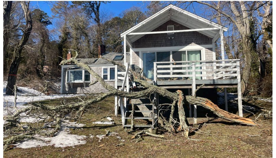
This damage from February 2026 storm highlights the danger of the invasive black locusts, whose shallow root systems and brittle wood can lead to uprooting and broken limbs.
