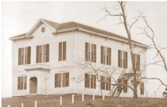
Figure 3. 1928 view of Orleans Town Hall.
